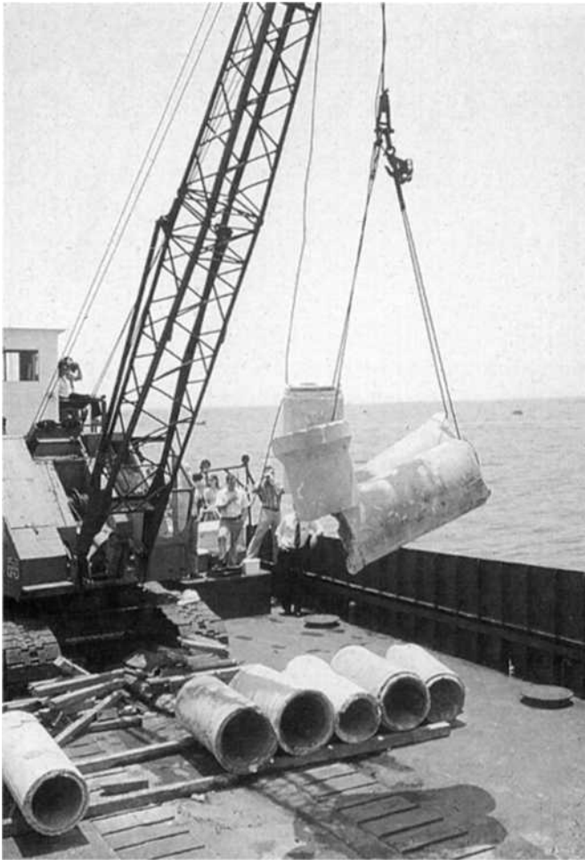
Scientists place culverts in the Gulf of Mexico for the Pinellas County Reef Program.
